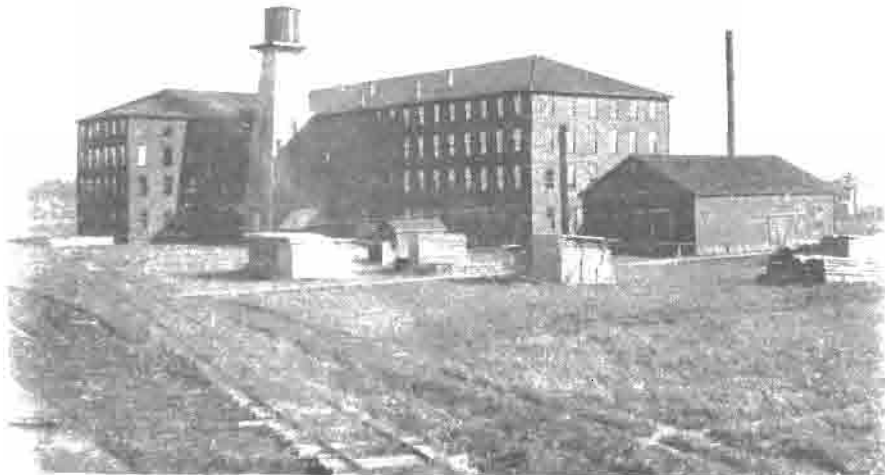
The Carriage factory at 13th and A streets.
